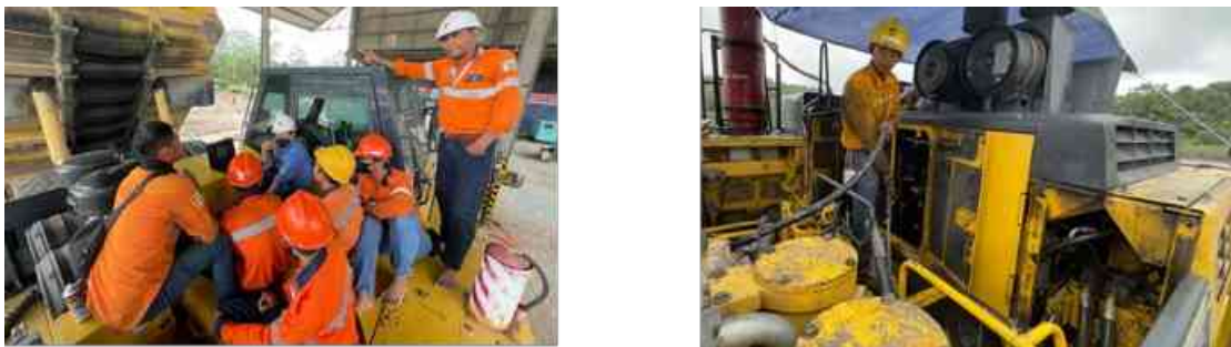
Figure 4.9 Procces Replacement Hose PC1250-8 in Hydraulic System
